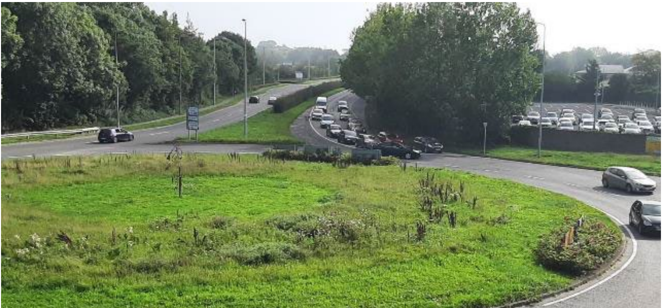
Diagram 27.14: Seatown Road Roundabout and R132 Looking Southwards from Footbridge at Woodies Car Park
