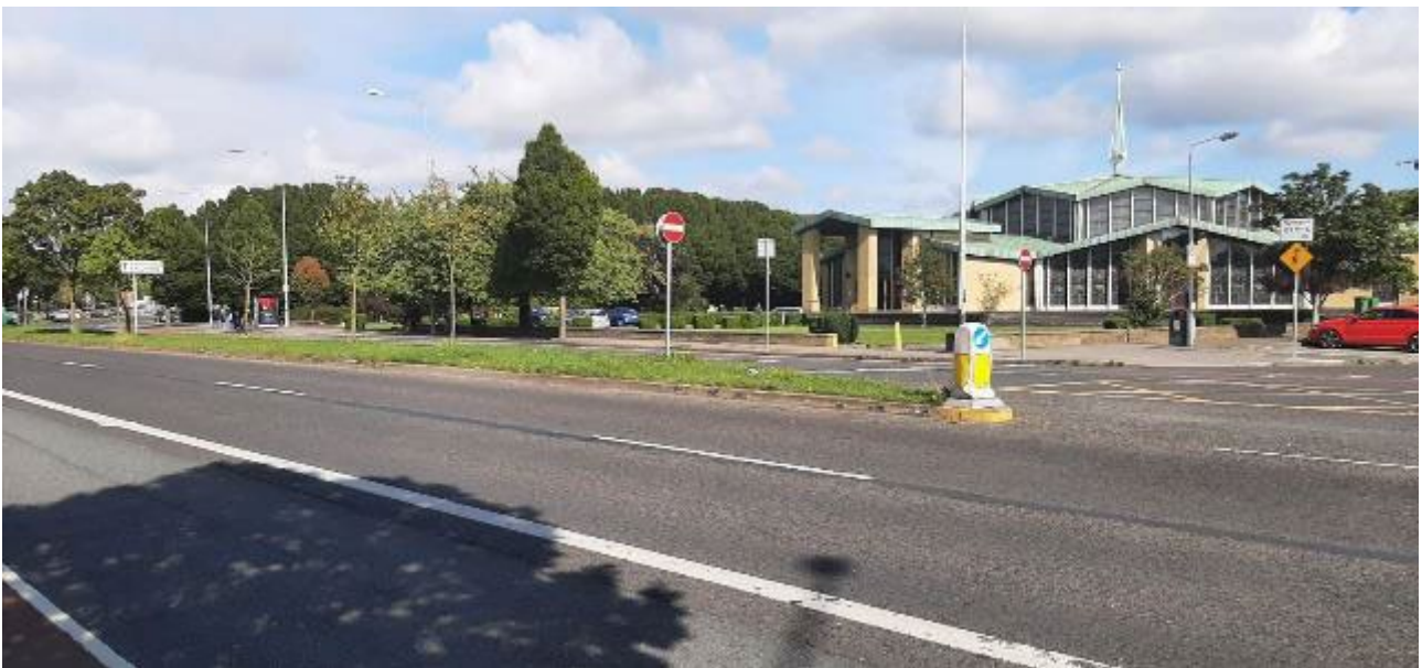
Diagram 27.35: Our Lady of Victories Church Beyond the R108 Ballymun Road Looking North-East
