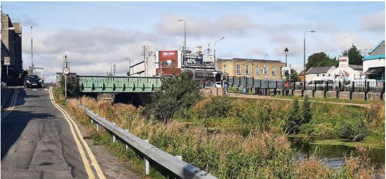
Diagram 27.43: Looking North-West from Eglinton Terrace Towards Cross Guns Bridge and the Proposed Glasnevin Station Site Beyond
