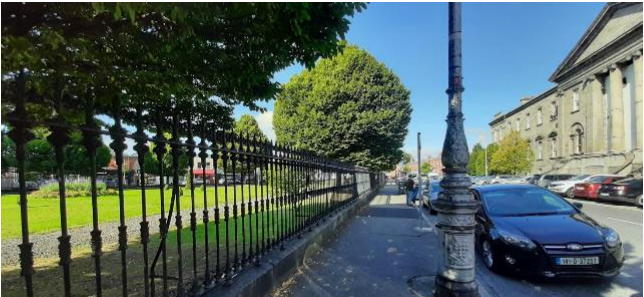
Diagram 27.47: Existing View from Eccles Street with the Railings to the Park and the Mater Hospital Building on the Right
