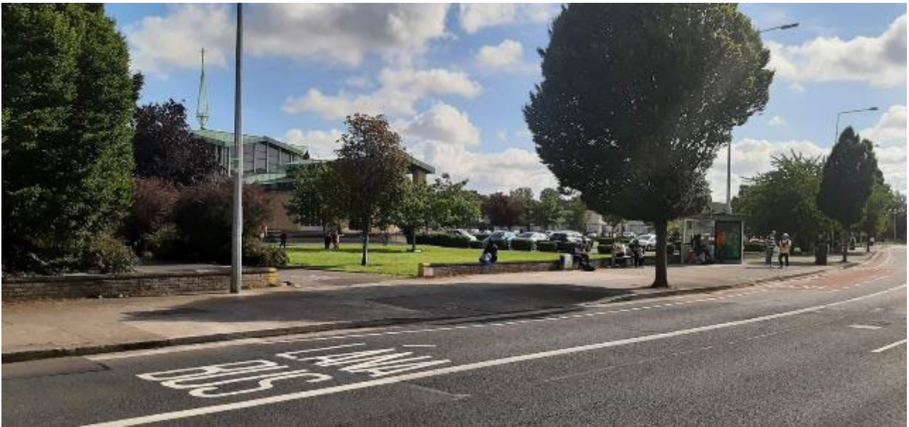
Diagram 27.34: Our Lady of Victories Church Beyond the R108 Ballymun Road Looking South-East
