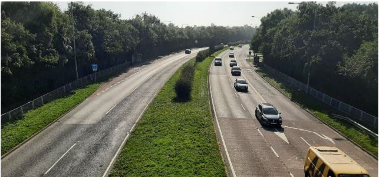
Diagram 27.17: The R132 Southwards from 'Pavilions' Footbridge at Malahide Road Roundabout
